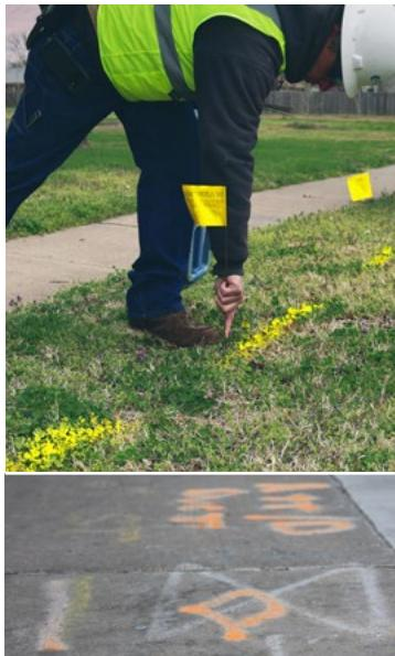
When a construction project is planned for a specific area, line locators mark underground facilities so excavators know not to dig near the markings. While it may just look like a mess of lines, “utility graffiti” is a very important safety precaution; and unlike other graffiti, these utility markings will fade after a few weeks.
